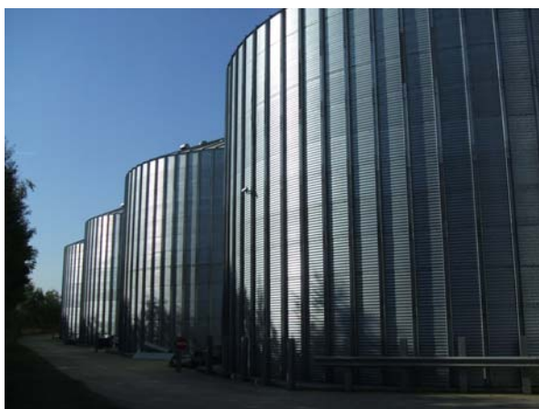
Plate 3. Trial silos containing 3, 000 t of wheat at Cambridge store.
