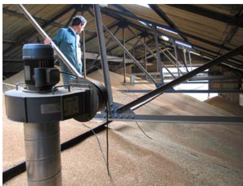
Plate 2. Pedestal ducts and view across Darlington store (700t wheat).
